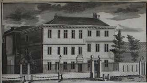
View of The INDEPENDENT ACADEMY, at HOMERTON, near Hackney.
